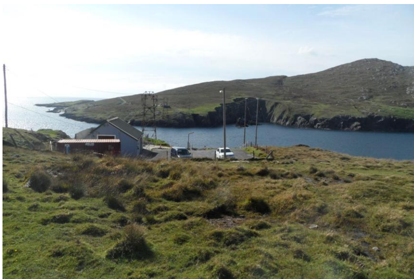
Plate 3.14: Car park at Garnish View.
