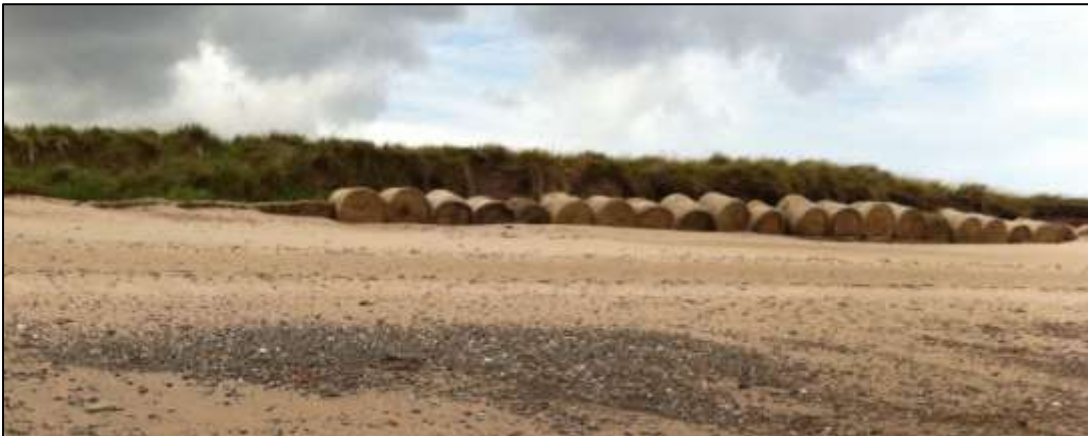
Figure 3.15 Bales being used to manage erosion of dunes on Castlegregory beach
