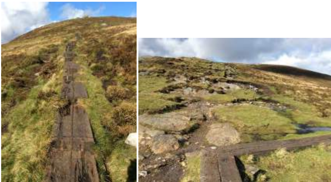
Fig. 9 Constructed path made from railway sleepers on approach to the JB Memorial Stone and shortly before the end of the constructed boardwalk where walkers start their final ascent up to the summit of Djouce from the western side.
