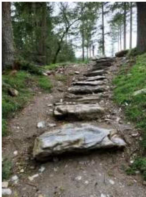
Fig. 25 Stone steps on path not performing their expected role.
