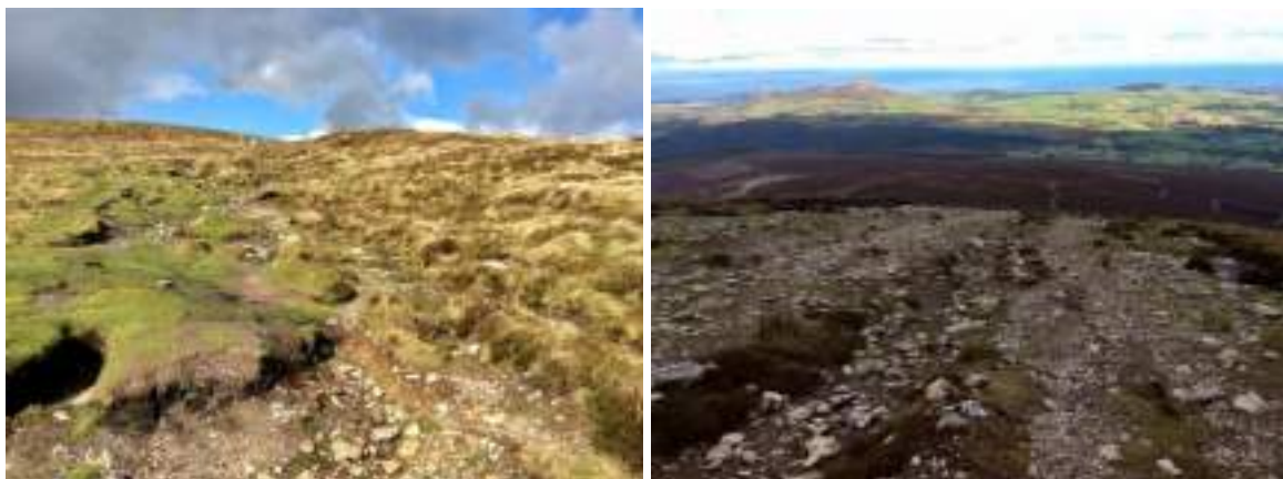
Fig. 12 Lateral erosion on both the western and eastern approach to the summit.
