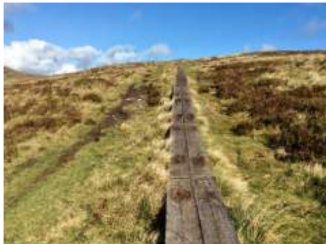
Fig. 10 Eroded parallel path to the boardwalk evident made worse by mountain bikers spilling out from Ballinastoe MTB Trail Centre
