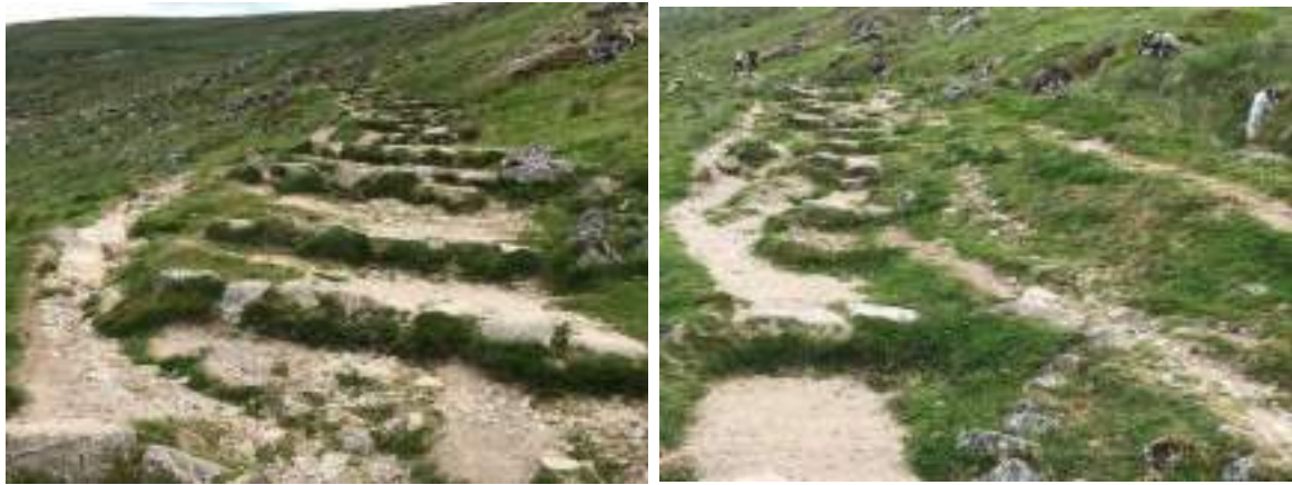
Fig. 24 Lateral erosion causing damage to the soils and vegetation as walkers take a more comfortable detour around the original stepped path
