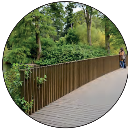
New bridge across water course
