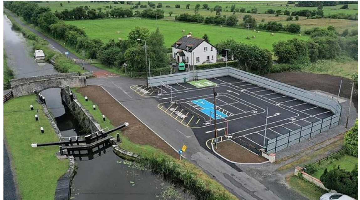
Car park on the Grand Canal Greenway at Cappincur
