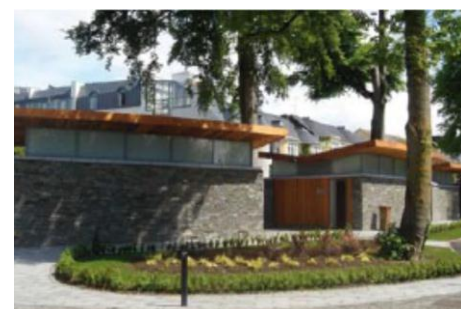
Killarney Public Toilets: Well designed and well maintained.
