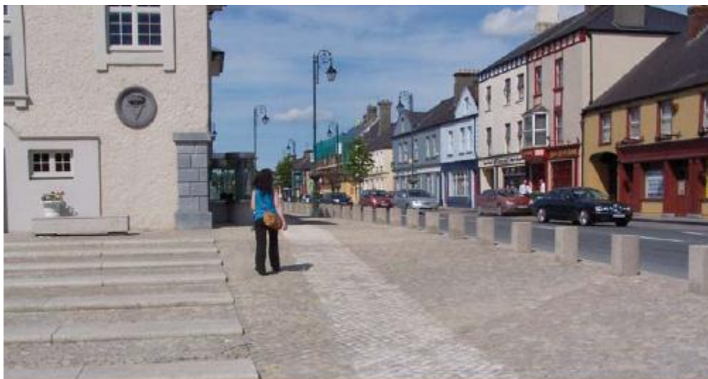
Abbeyleix, Co. Laois: New paving outside the restored Market House, now a County Library. The building is located on a crescent shaped open space, which is re-paved to create an attractive area, separated from the main road by stone uprights as bollards.
