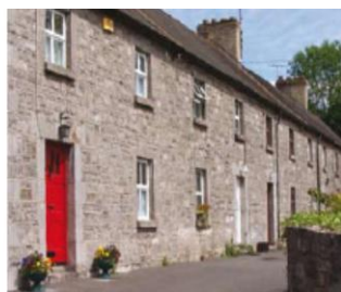
Mill cottages in Slane have beautiful cut stone surrounds flush with coursed stonework, with overhanging slate roofs. Traditional buildings like this are intrinsic to the particular character of Slane.
