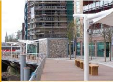
Clarion Hotel frontage onto the River Lee, reinvented to provide out of doors space under cover and car park access. The timber board is an extension to the quayside.
