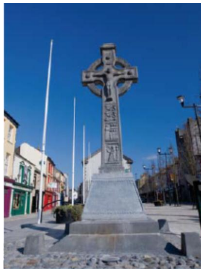
Improvements for pedestrians in Cashel Town: Note the new lighting stands, trees, paving and signage, and the removal of overhead wires.
