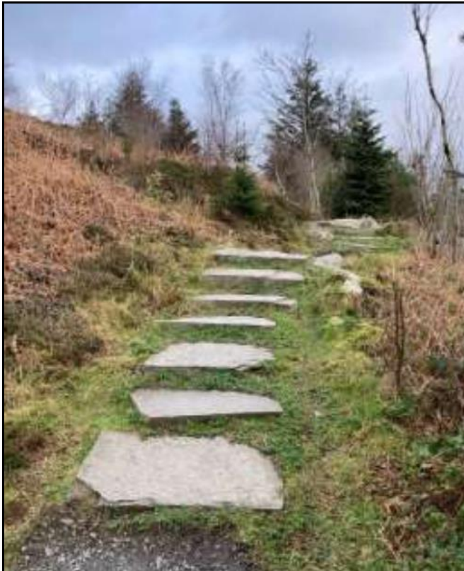
Figure 5.3: Example of stone stepping proposed for 18% of Trail
