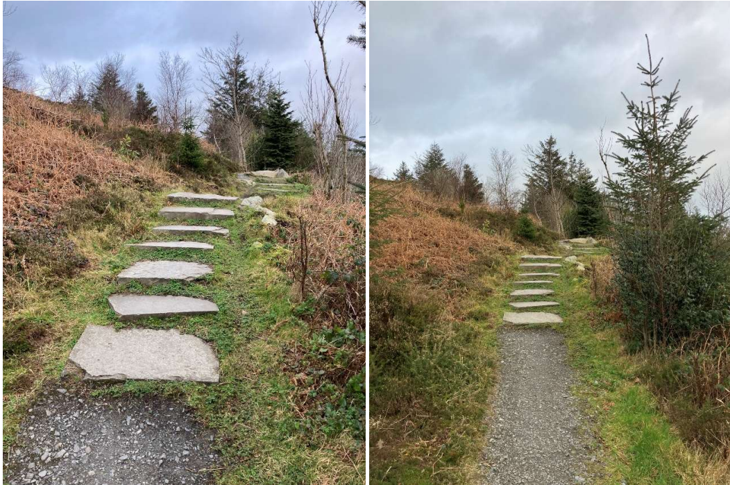
Figure 22 Example of stone stepping with gravel sections to accommodate gradient incline
