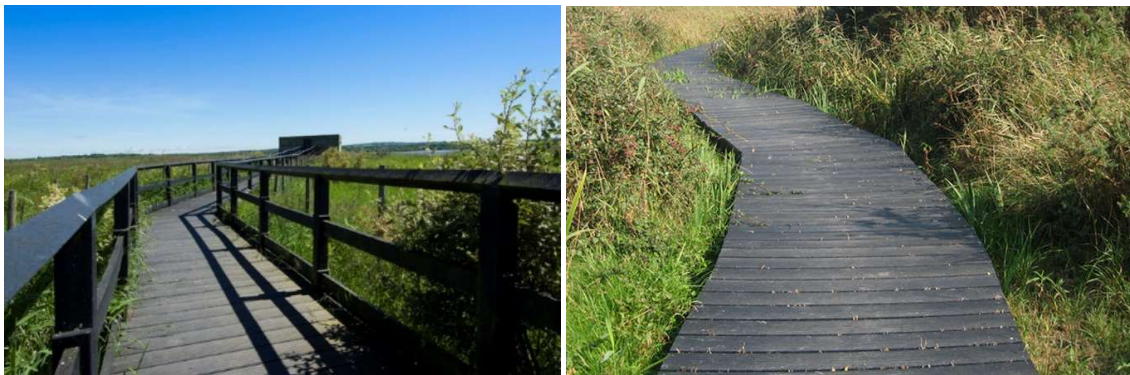
Figure 21 Examples of recycled plastic boardwalk, with and without handrails
