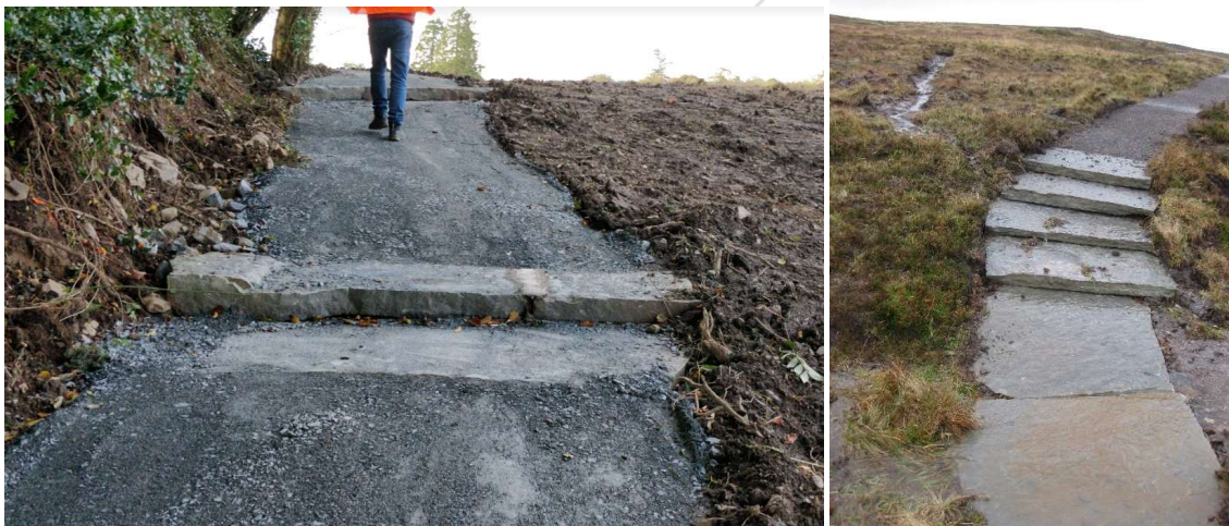
Figure 25 Anchor stone stepping with gravel trail and stone stepping with gravel trail
