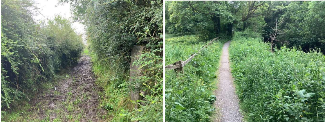
Figure 11 Trail requiring new build gravel trail, section of existing fit for purpose trail
