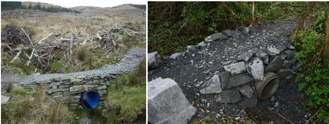
Figure 32 Examples of culverts with twin headwalls
