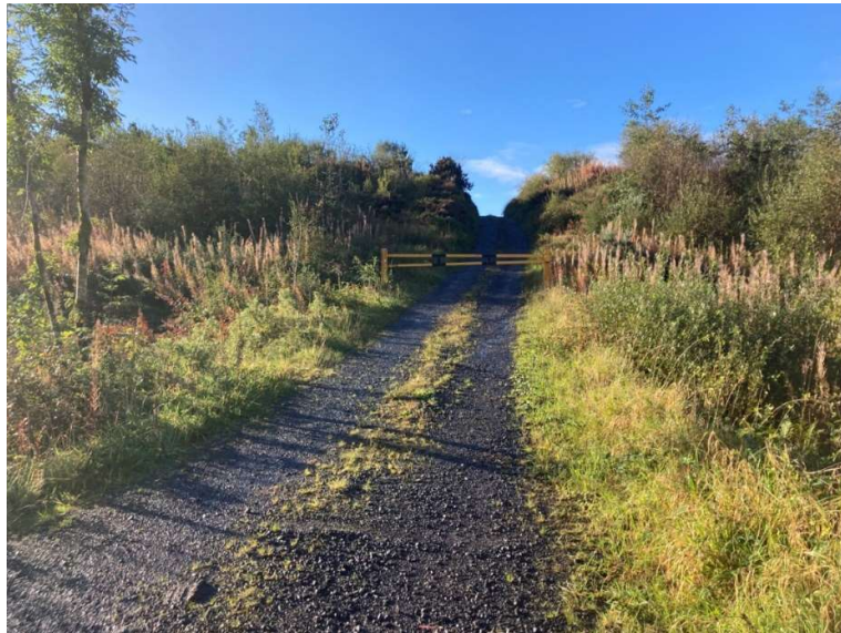
Figure 21 Example of vehicular access hardcore section on BBW
