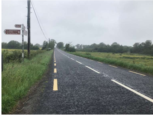
Figure 5 Section of bound surface, on road trail - Lung Lough Gara Way
