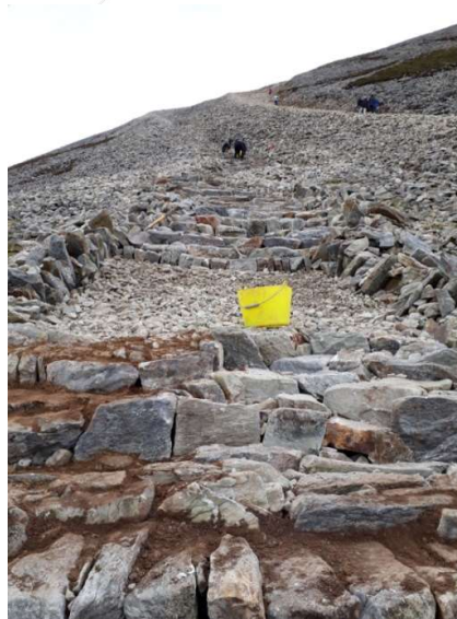
Figure 29 Scree pitching in progress on Croagh Patrick
