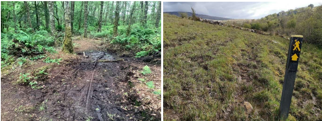
Figure 17 Sections requiring new build trail with geotextile
