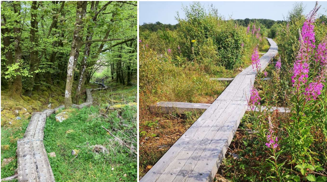
Figure 19 Example sections of bog bridge - Cavan Burren Park and Scohaboy Bog
