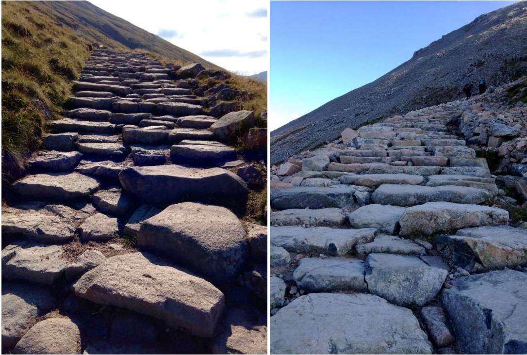
Figure 28 Examples of classic stone pitching in upland environment
