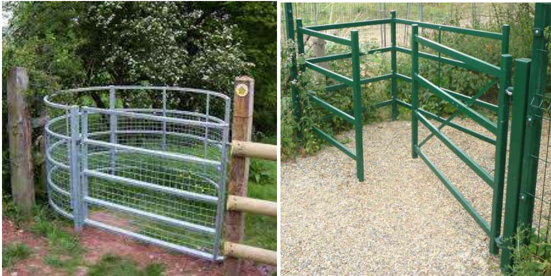
Figure 41 Kissing gate, curved enclosure and rectangular enclosure
