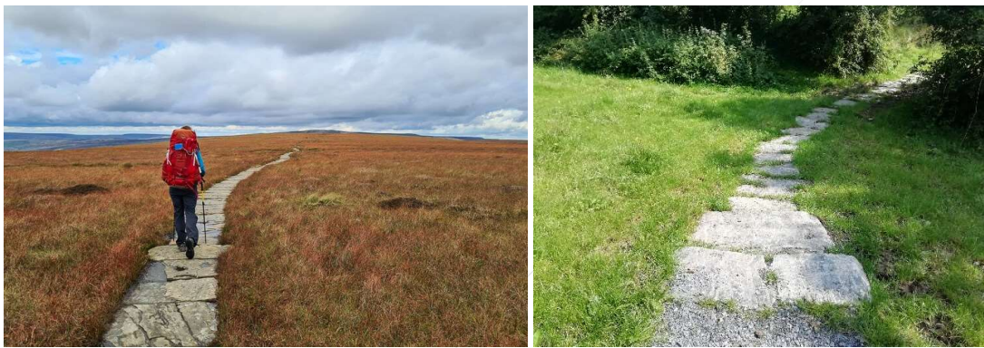
Figure 26 Flagstone paving on the Pennine Way (© Becky Angell) and continuous stone stepping
