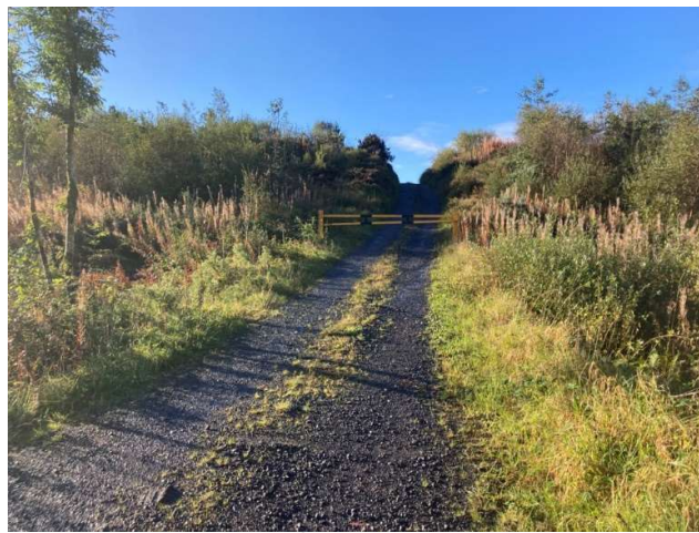
Figure 4 Existing section of unbound hardcore vehicular access trail - no works required
