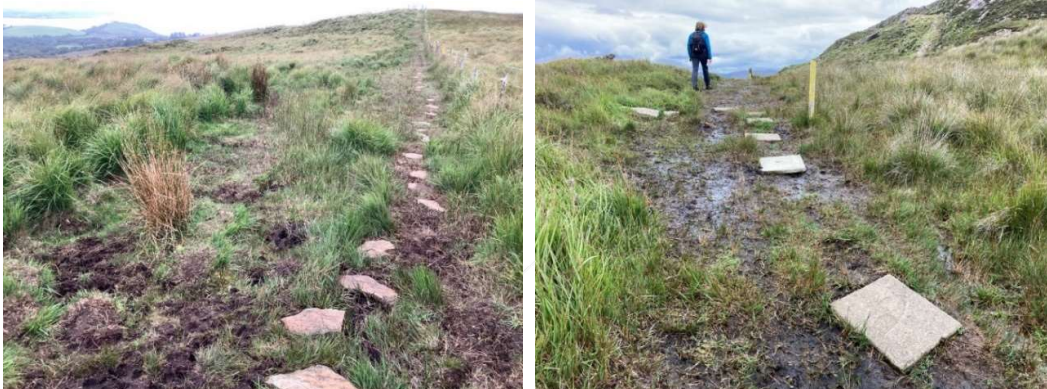
Figure 2 Use of stepping stones to traverse wet areas
