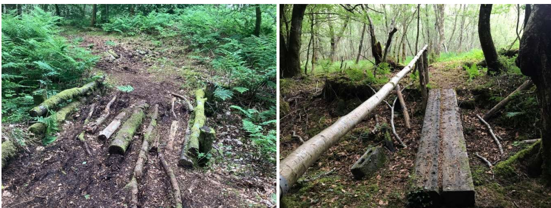
Figure 31 Infrastructure not fit for purpose on the Suck Valley Way
