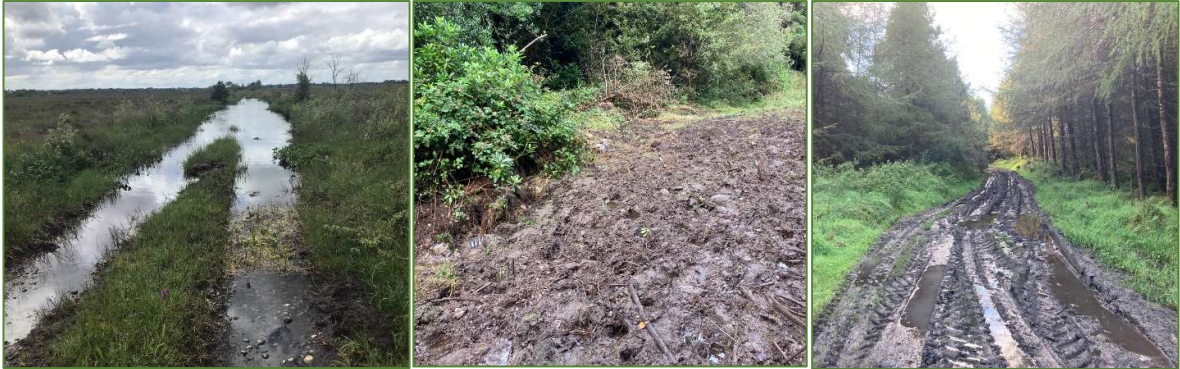
Figure 9 Poor condition trail - standing water, badly poached, damaged by vehicles
