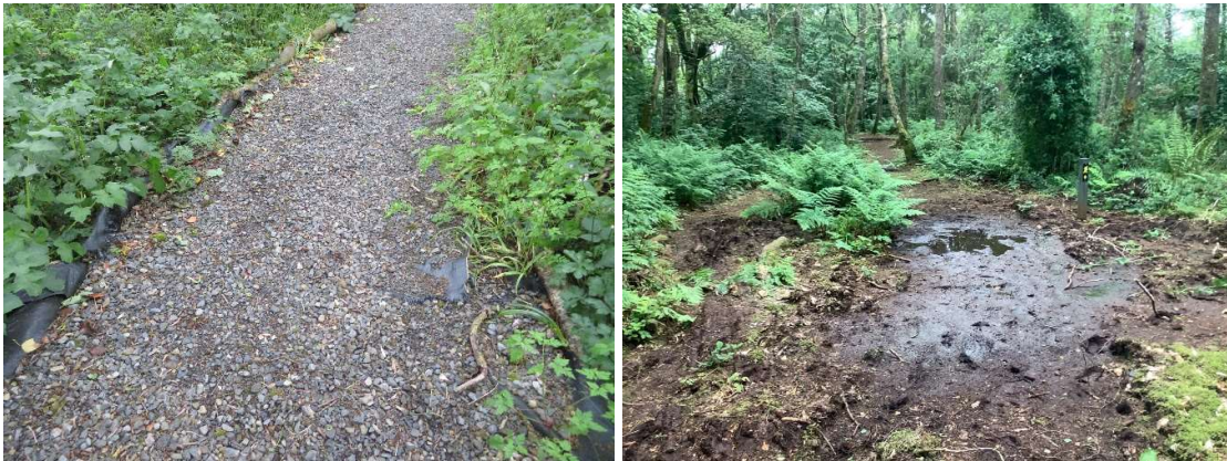
Figure 30 Trail in poor condition on the Suck Valley Way
