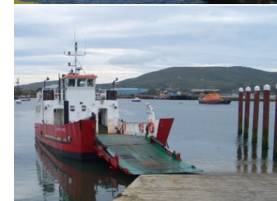
Types of Infrastructure From top to bottom - pontoon; pier with steps;
